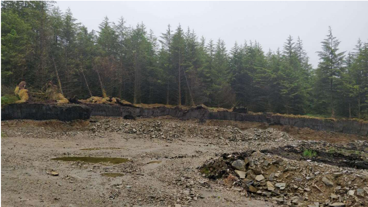
Figure 6-3: Ground conditions observed along route C
