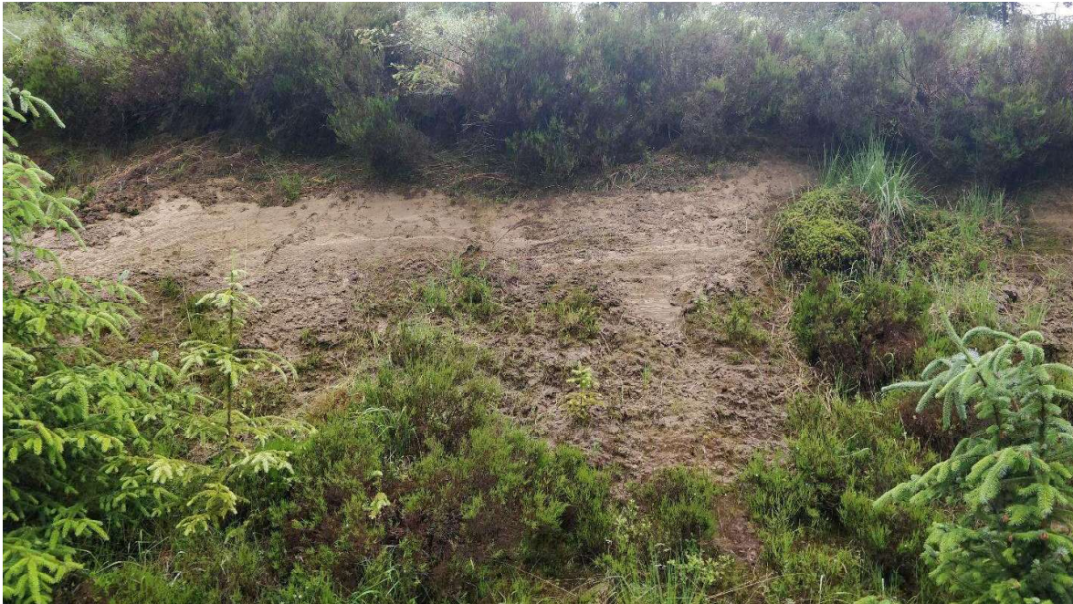
Figure 6-6: Exposed overburden cut with evidence of erosion/shallow slips (ITM 516203E, 582880N)
